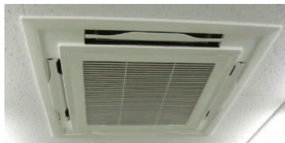
Inverter type air conditioning facilities
